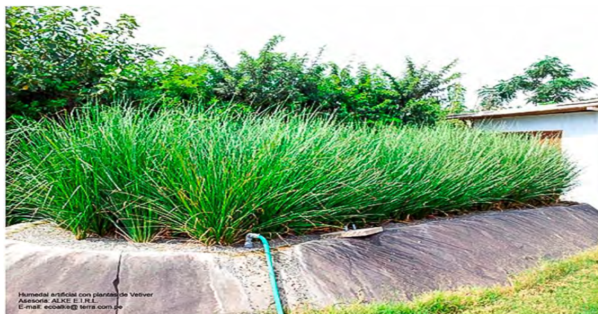
Treatment plant of domestic waste water with vetiver plants in a private home in Lima (20m 2 ),.
